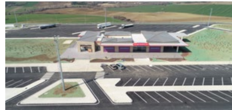
Lapseki Otoyol Hizmet Tesisleri. Lapseki Motorway Service Area.
