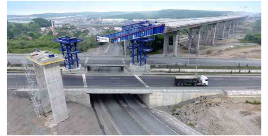
KMO-2 İhsaniye Viyadüğü İtme Sürme-Ardgerme. NMM-2 İhsaniye Viaduct Incremental Launching and Post-Tensioning works.
