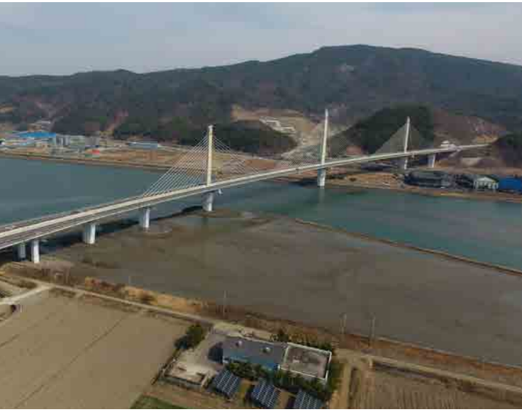
Çapraz kablolu kavisli gergi askılı Sepung Köprüsü. Curved cable-stayed bridge with transversal cables, Sepung.
