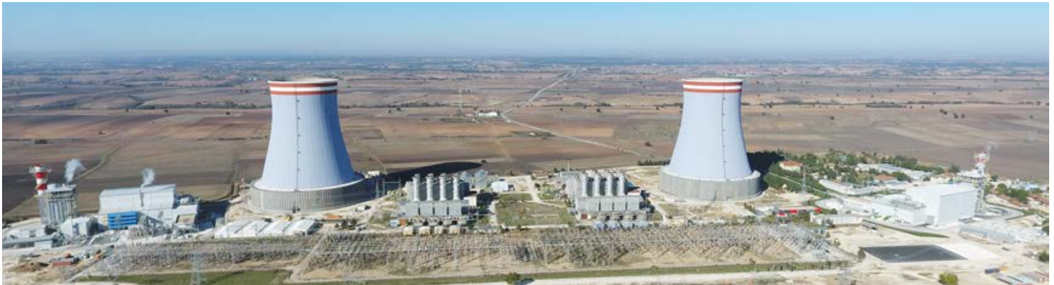
Hamitabat Natural Gas Combined Cycle Power Plant
