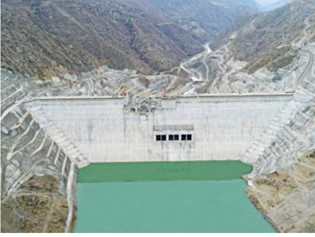
Siirt Çetin Barajı Siirt Çetin Dam
